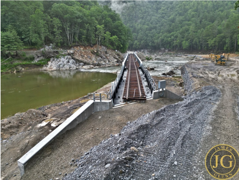
At left, the CSX Poplar bridge reconstruction has been completed. [James Glenn photo.]
