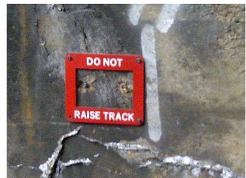
very crucial information regarding track height and the limit to which track can be raised by the engineering department. If this tag is read wrong, and the track is pulled too high, then we risk shaving off the top of a doublestack container and costly repairs to the bridge and track. Autorack cars present a two fold problem. If you have ever paid attention to a typical autorack car, you have noticed the hundreds of fifty-cent piece sized holes that line up in rows across
