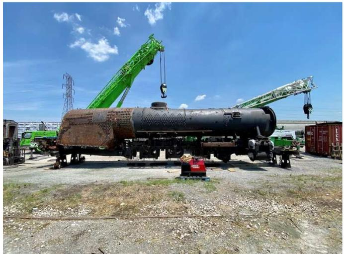
removed one at a time. Each driver wheel was dragged using a telehandler rather than rolled due to the lack of side rods acting as a balance to the counterweights. The engine was then lowered onto four steel pedestals. The driver wheels will be sent to the Tennessee Valley Railroad Museum in Chattanooga where they have the special machinery needed and FMW Solutions will perform the repairs and needed maintenance.
