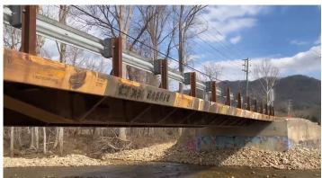
Petal, Mississippi-based IBC has so far installed more than 40 railcar bridges in seven counties.
